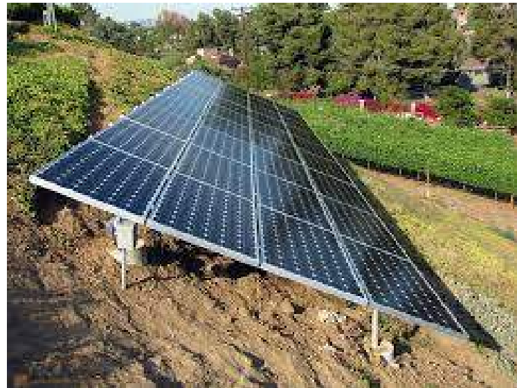
GROUND MOUNTED PV PANELS ON SLOPE
